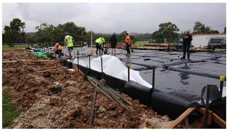
Work continues, still working on the membrane - a lot of sealing to be done on the corners of each of the sand blocks.
