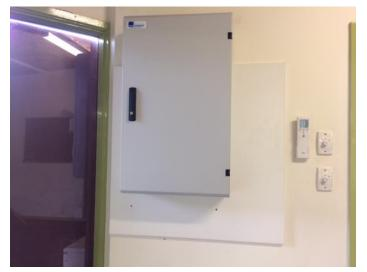
New switchboard installed by council with the fan switches outside of the board.
