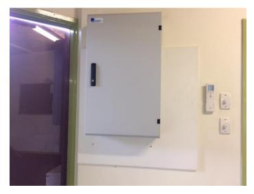
New switchboard installed by council with the fan switches outside of the board.
